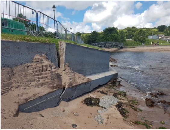
Structural Failure and Scouring Evident
