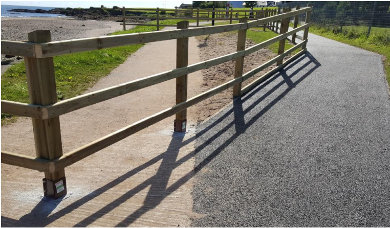
Footpath Relocated and Area Made Safe
