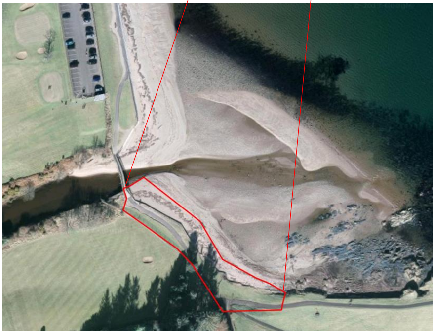
Location of Failure
