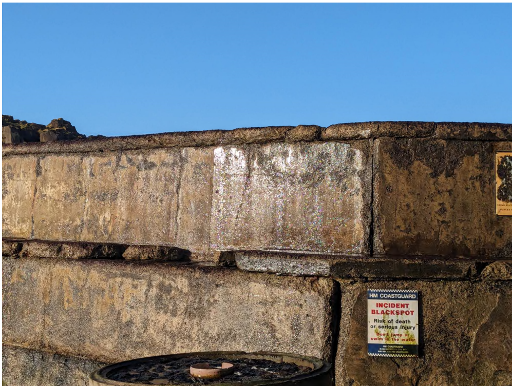
Portions of concrete parting with original cast in-situ structure
