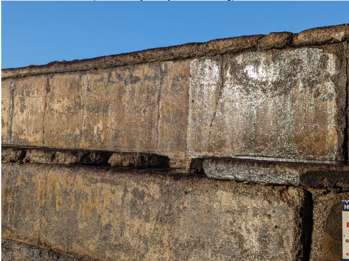
Portions of concrete parting with original cast in-situ structure
