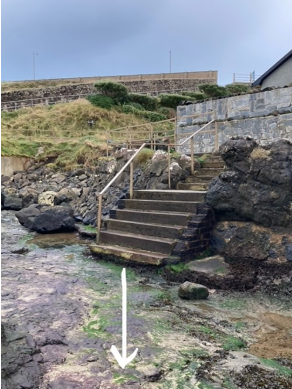
Photo B – New path location from existing steps onto rocks
